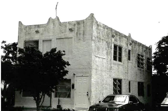
Photo of 518 South L Street provided in the 2002 Florida Master Site File
